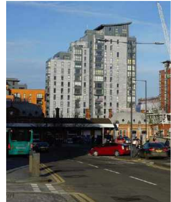
CLOCKWISE FROM TOP: View towards Slough town centre across Lascelles Park; Lexington apartments to the north of the railway station; and St Mary's Church
